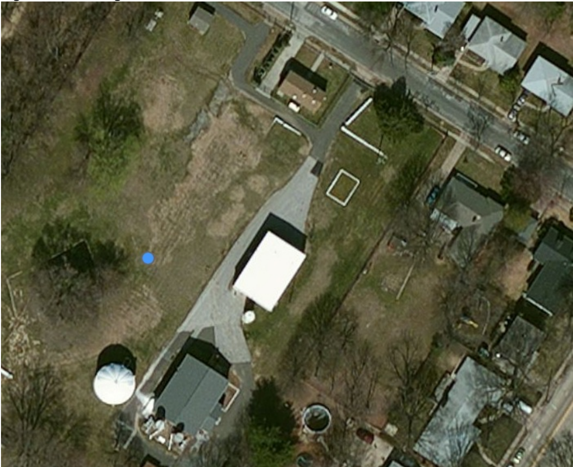
Figure 1: Browning Road Water Treatment Plant
