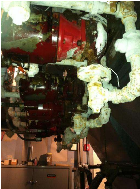
Picture: AC-1 Zone Reheat Coils
