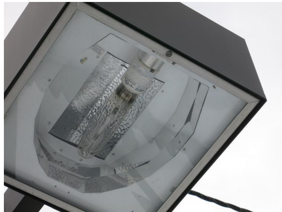
Image 16: 240W Sodium Vapor Exterior Lamp
