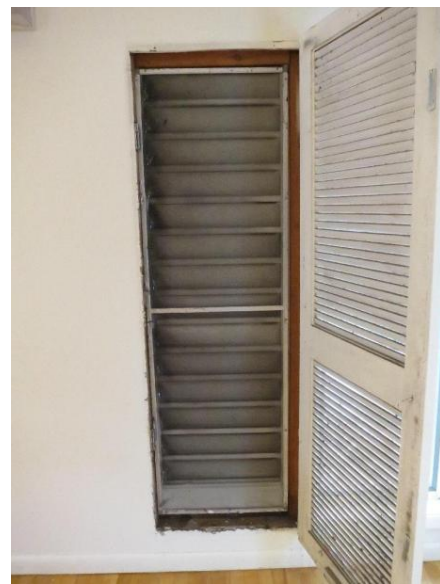
Image 3: Ventilation Structure in Anderson Auditorium
