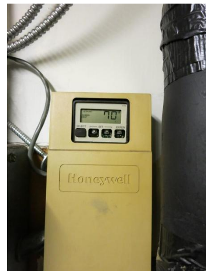
Image 12: Thermostat in Basement Classroom Image 13: Temperature Control for Boilers
