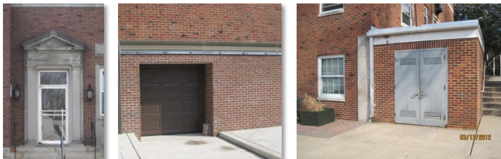
Typical door types with no visible energy-compromising issues
