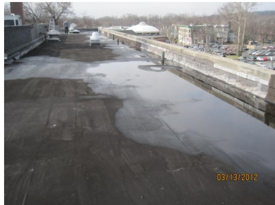
Signs of improper drainage and standing water
