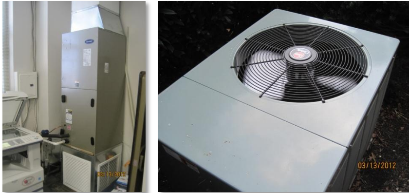
Indoor cooling fan coil unit with corresponding outdoor condenser
