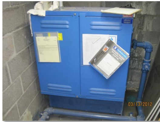
Submerged hydraulic type elevator motor
