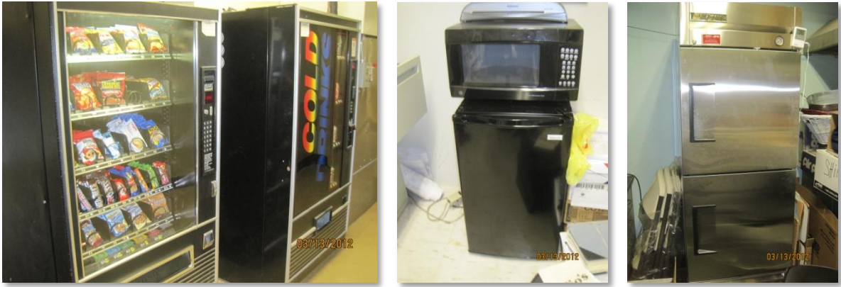
Typical plug-load appliances located throughout the building
