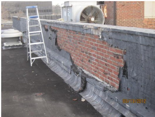
Decayed and peeling sealant
