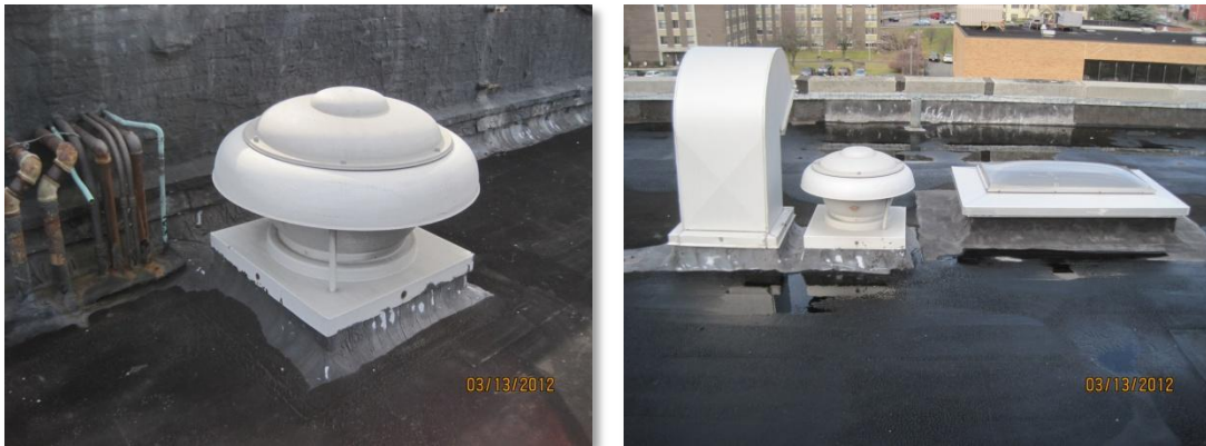
Typical rooftop exhaust fan units
