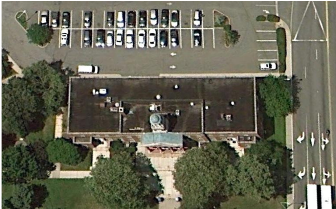
Satellite image of the Municipal Building courtesy of Google Earth
