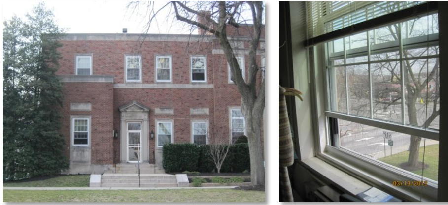
Typical single-hung window units and a transom unit over the glass door. Units exhibit no signs of energy-compromising issues.
