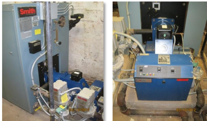
Gas-fired Steam Boiler located in basement Boiler Room
