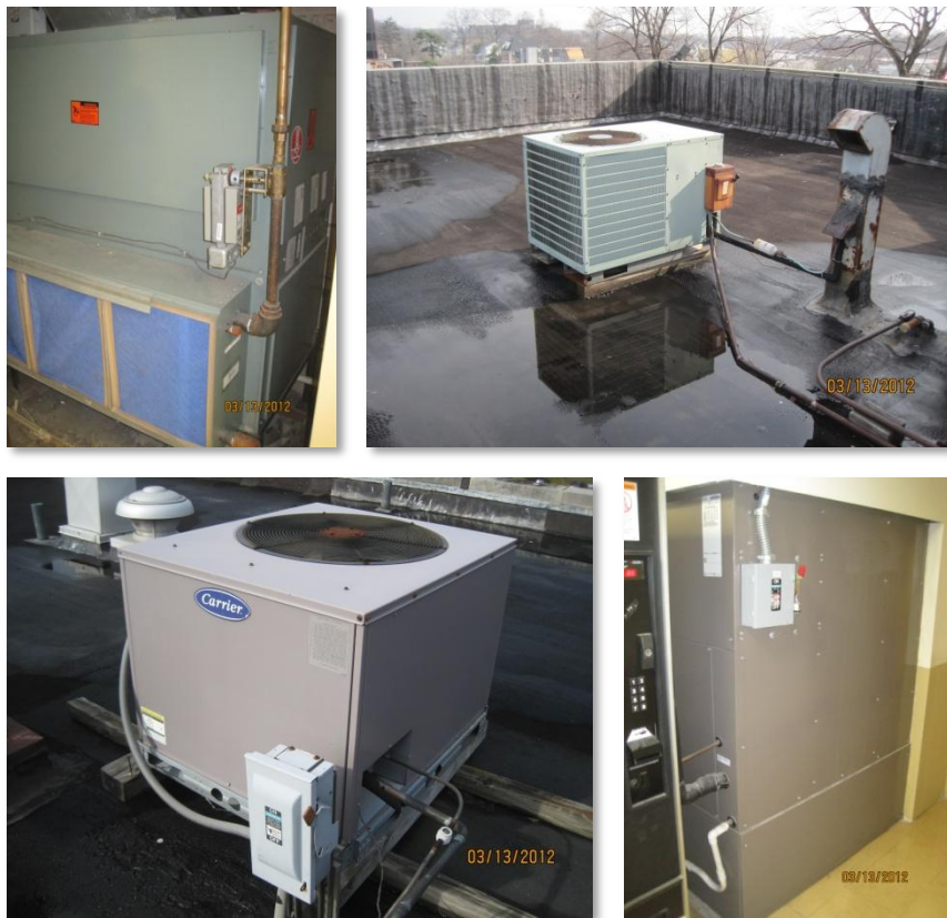
Typical air handling units with corresponding rooftop condensers
