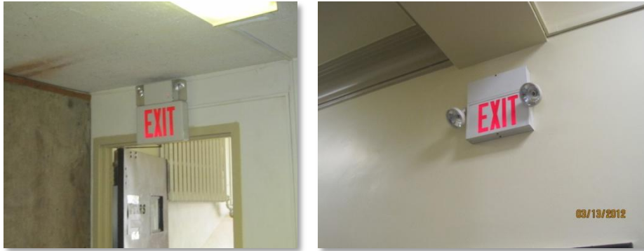
Typical LED exit lighting
