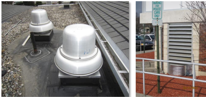
Typical rooftop exhaust units and louvers
