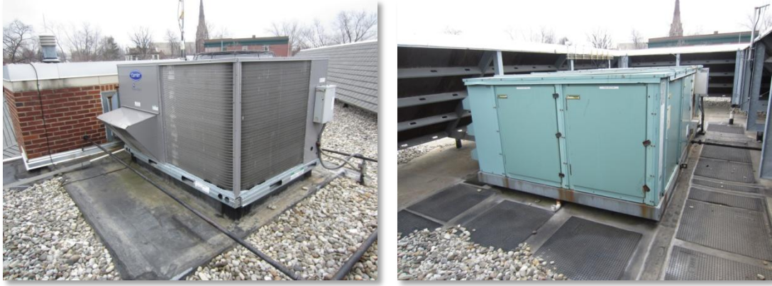
Typical packaged rooftop units
