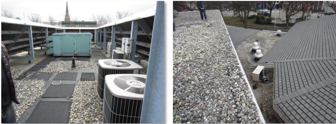
Typical roof system with no visible energy-compromising issues
