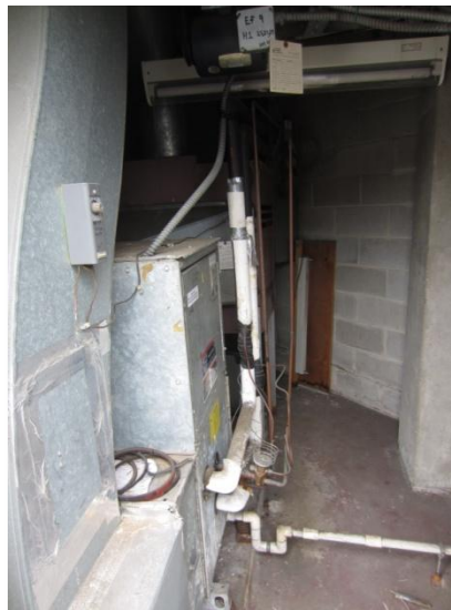
Carrier air handling unit
