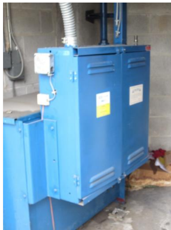
Submerged hydraulic type elevator motor
