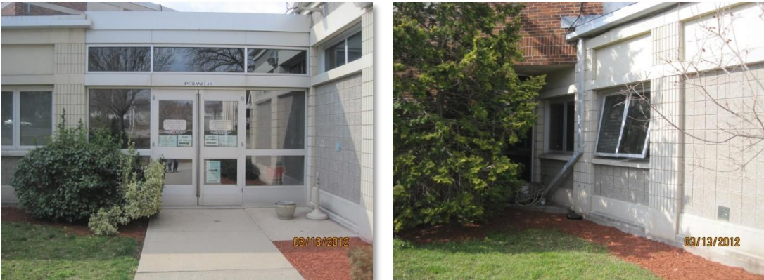
Typical transom and awning windows with no visible energy-compromising issues other than the non-insulated aluminum window frames.
