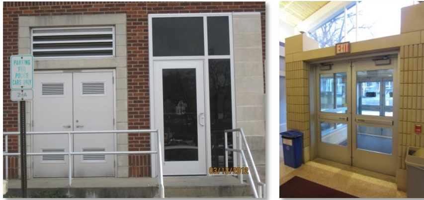
Typical doors with no signs of energy-compromising issues
