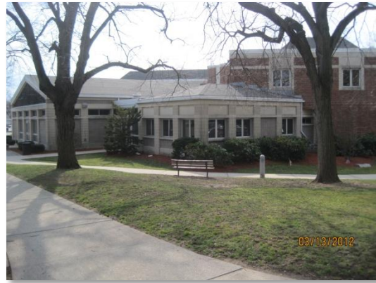
Partial North Façade
