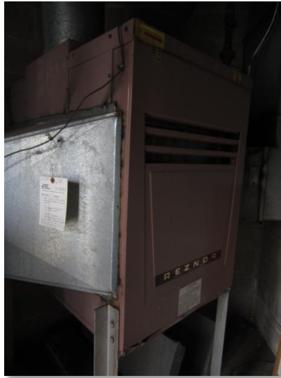
Reznor gas-fired unit heater
