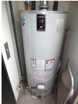
Natural gas-fired domestic hot water heater
