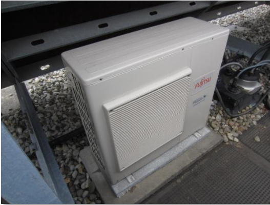
Split system units and corresponding rooftop condensers
