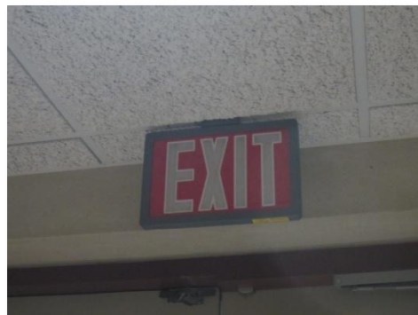
Typical photoluminescent LED exit lighting
