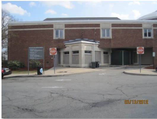
Partial West Façade
