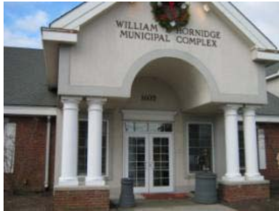
Brick masonry exterior walls with EFIS near vestibule
