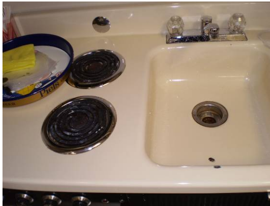
Kitchenette sink with flow measuring 4.5 gpm
