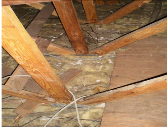
Wooden trusses with 6" batt insulation
