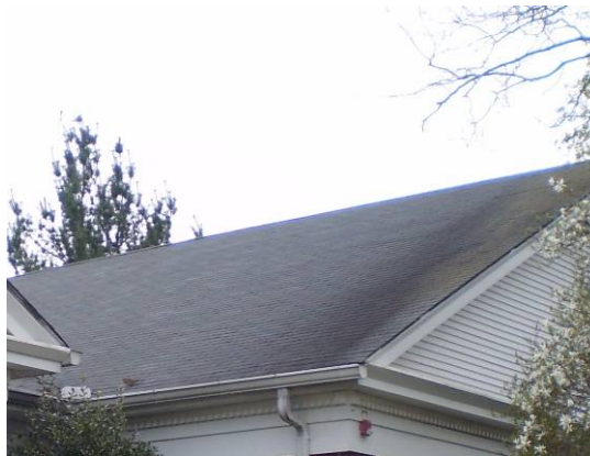
Asphalt shingles on pitched roof
