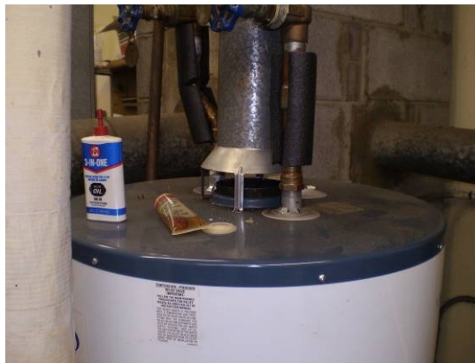
Atmospheric DHW Heater
