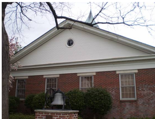
Face brick on lower portion; siding on trussed section
