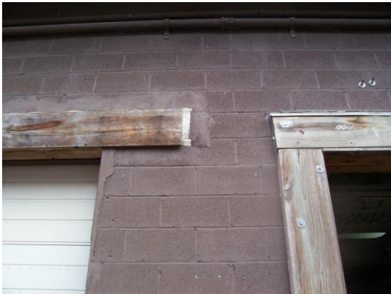
Signs of deterioration of the wood casings and a masonry rough spot were found
