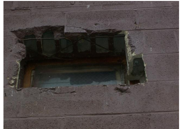
Signs of deterioration of the wood casings and a masonry rough spot were found
