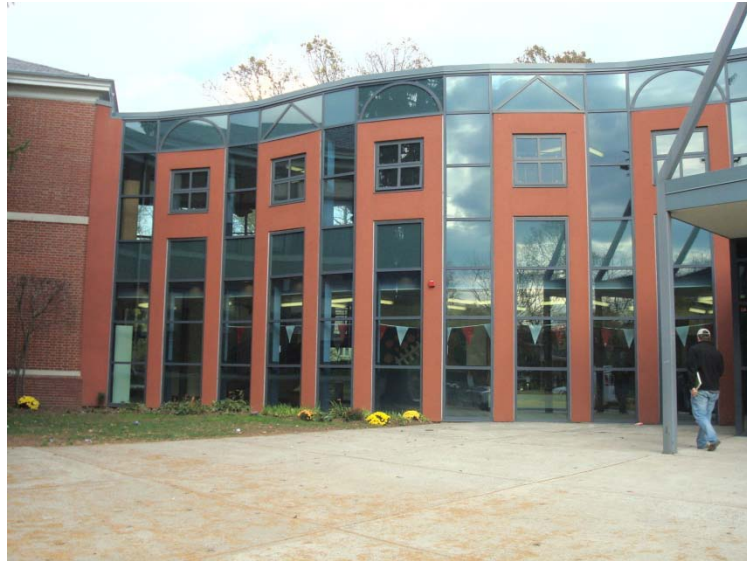
Example of typical installed windows
