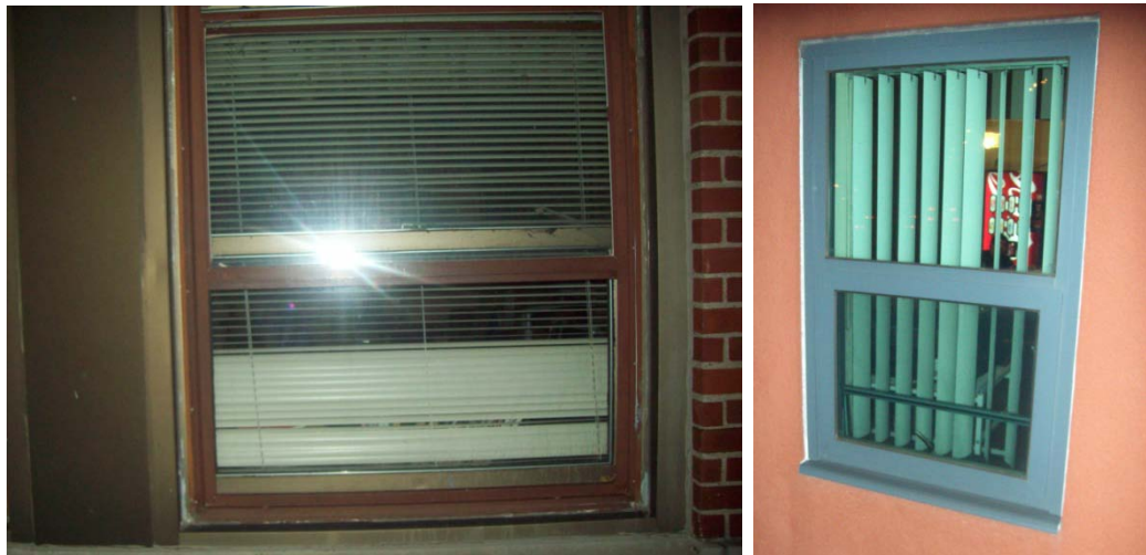
Examples of typical installed windows
