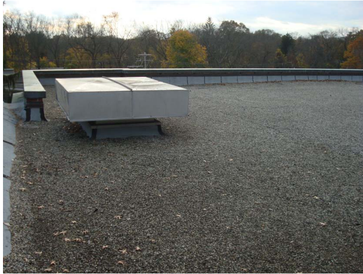
Example of gravel bed roof
