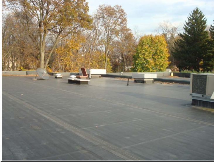
Example of EPDM flat roof
