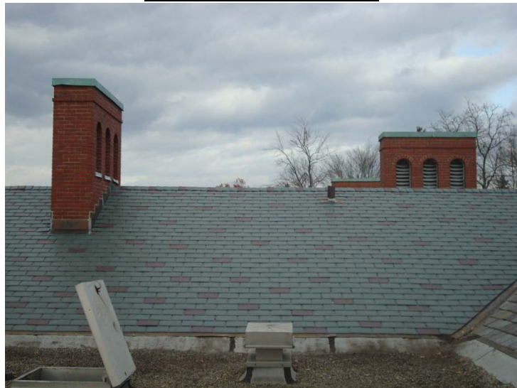
Example of sloped asphalt shingle roof
