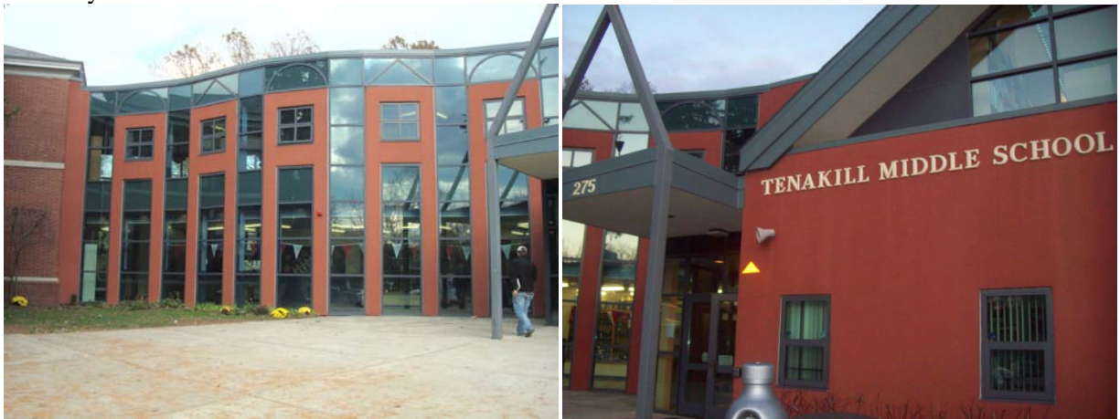
Existing Exterior Walls
