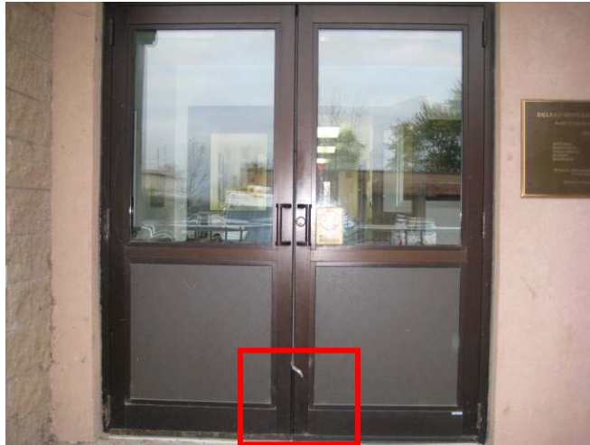
Control Building front door
