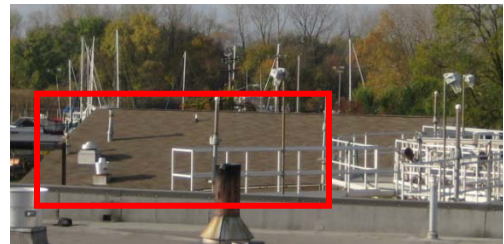
Roof in red box Control Bldg
