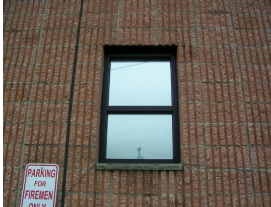
Typical Fire House Window
