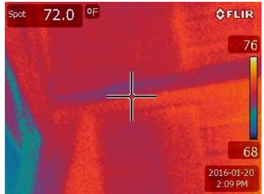
Exposed Timers colder than drywall
