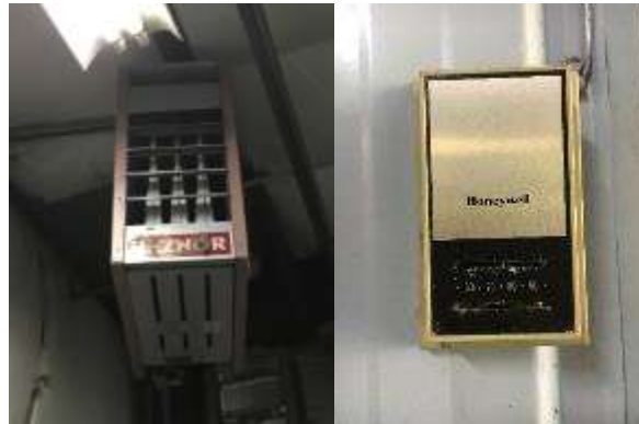
Image 4 – Gas Fired Heating
