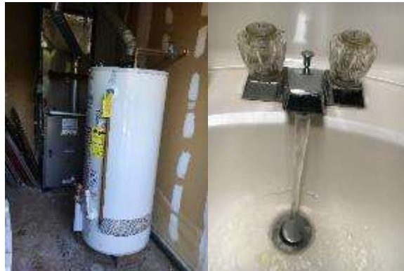
Image 3 – Domestic Water Heating
