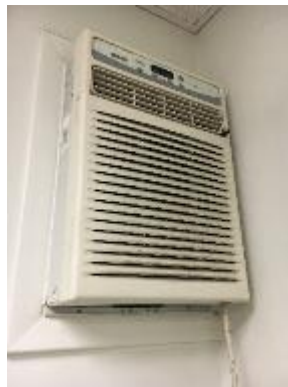
Figure 10 - Window AC Unit
