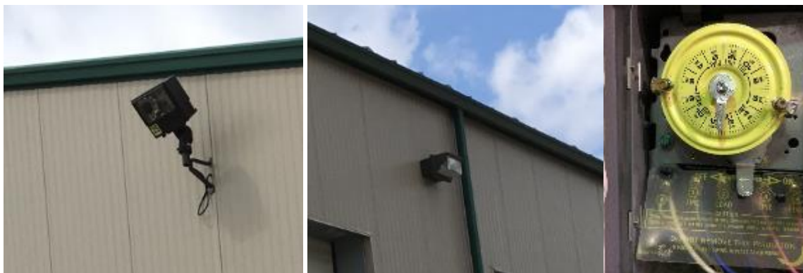
Figure 8 - Exterior Lighting and Timeclock Control
