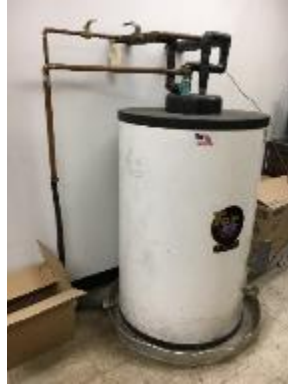
Figure 11 - Domestic Hot Water Tank
