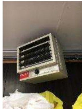
Electric HVAC equipment
