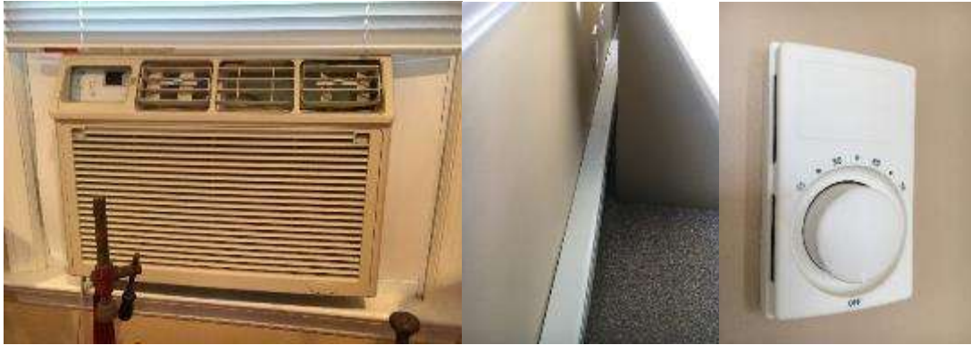
Image 3 – HVAC (Front Building)
