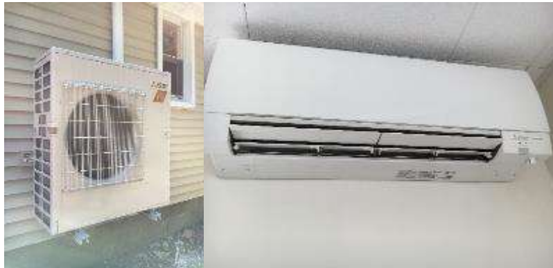
Image 4 – HVAC (Back Building)
