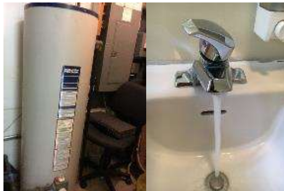
Image 3 – Domestic Hot Water
