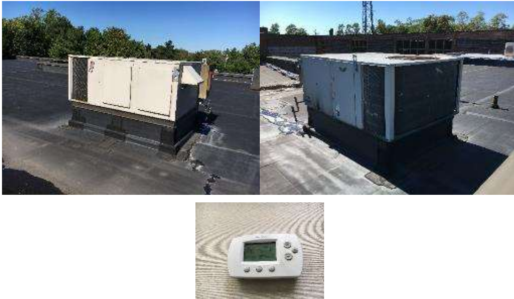
Image 5 – Rooftop Cooling and Controls
