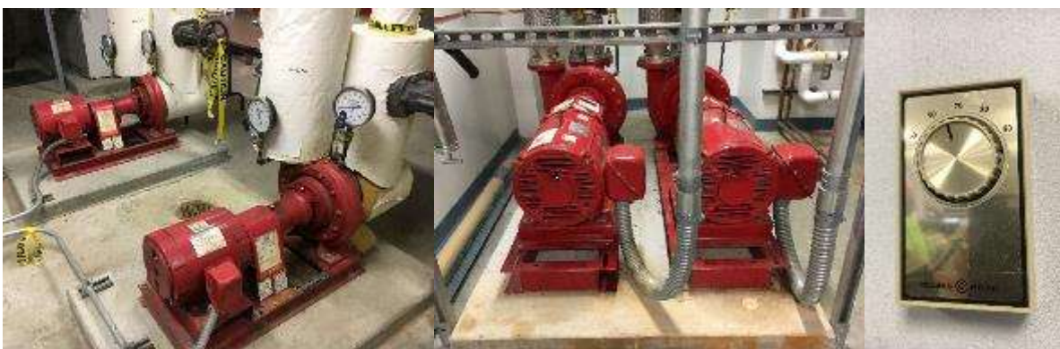
Image 4 – Heating Circulation Pumps
