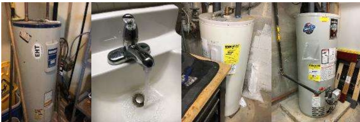
Image 7 – Domestic Hot Water
