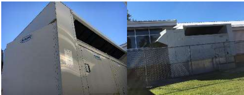
Image 3 – Air Handling Equipment - Economizers
