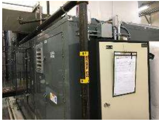
Image 2 – Package Air Conditioning Systems
