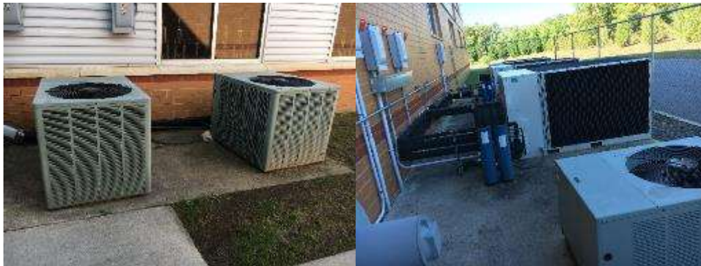
Image 4 – Condensing Units
