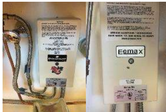
Image 6 – Domestic Water Heating
