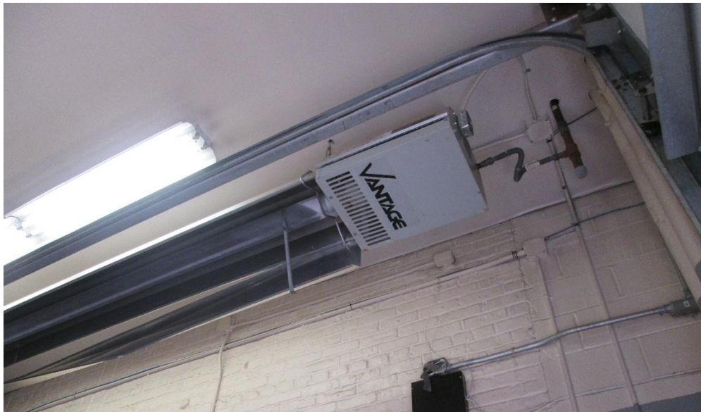
1. IR Gas Heating Unit
