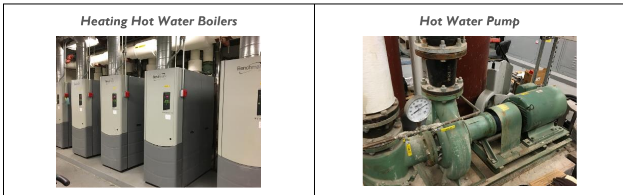
Figure 9 – Hot Water Systems
