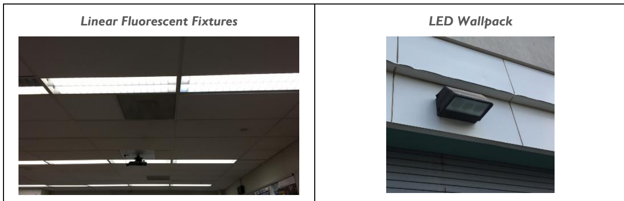
Figure 8 - Building Lighting Systems
