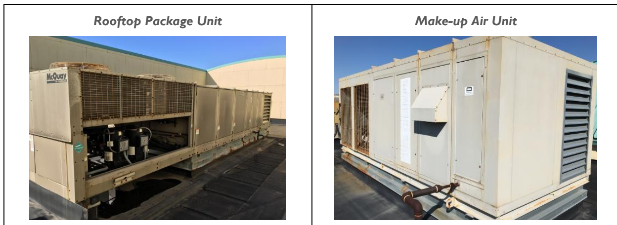
Figure 10 – Direct Expansion Air Conditioning Systems (DX)
