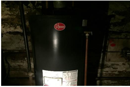
Rheem Fury (DHW unit in basement)
