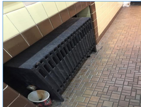
Radiator heating the dormitory
