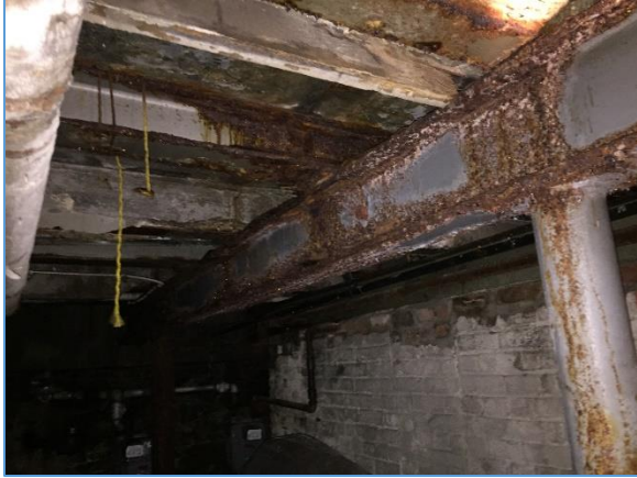
Corroded basement
