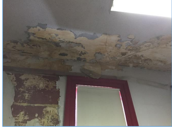
Ceiling with water damage
