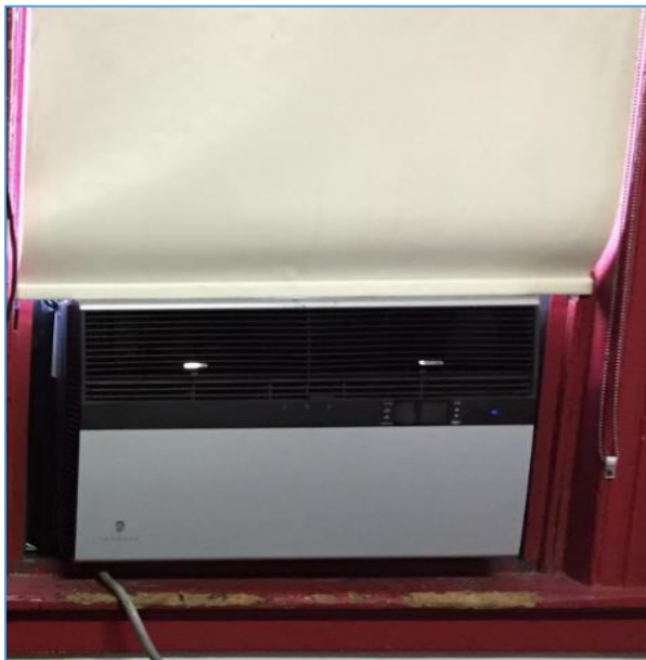
Window AC unit in the dormitory
