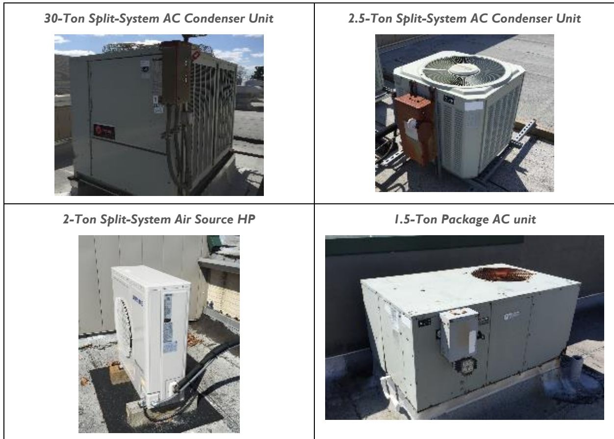
Figure 10 - Building AC Systems
