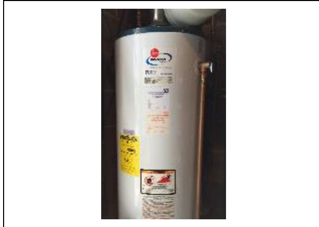
Figure 10 – Domestic Hot Water Heater
