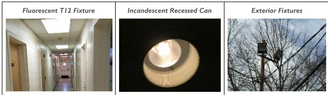
Figure 7 - Building Lighting Systems
