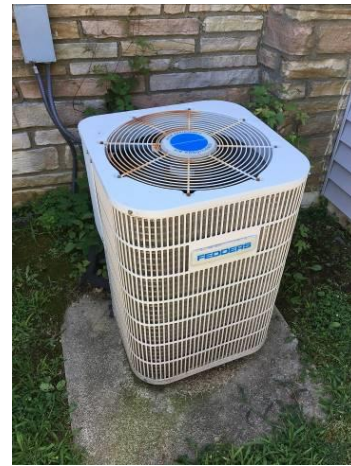
Annex Building – Condenser unit
