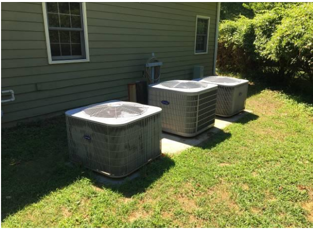
Nature Center – Condenser units
