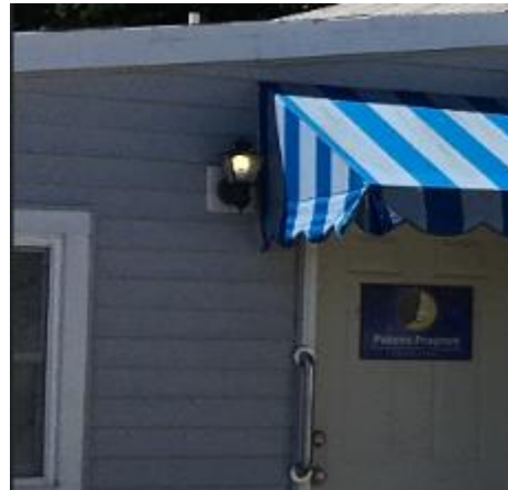
Annex Building– Entrance light (ON)
