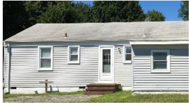
Annex Building siding, roof, windows, door
