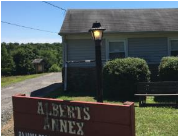
Annex Building– Pole light (ON)
