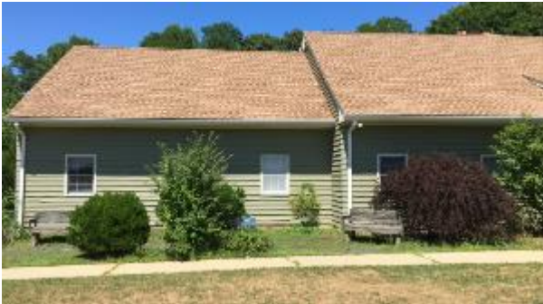
Nature Center siding, roof, windows
