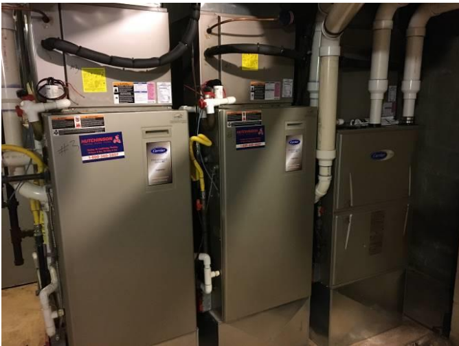
Nature Center – fan coil/furnace units
