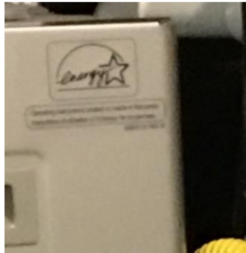
Nature Center – fan coil/furnace unit
