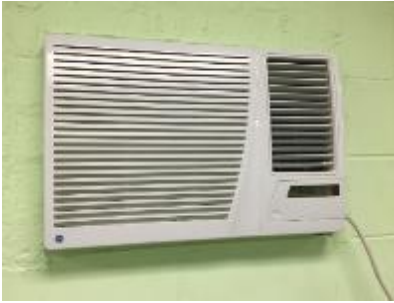
Image 11. Window AC Unit
