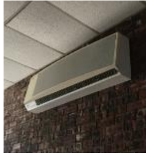
Image 12. Split System AC Indoor Unit
