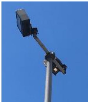
Image 8. Exterior Pole Mounted Fixtures
