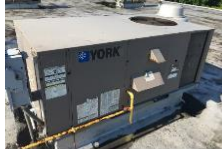
Image 13. Rooftop Package Unit
