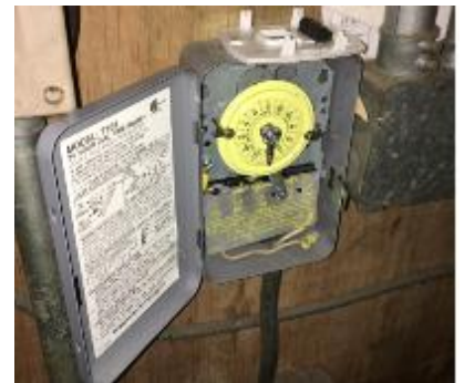
Image 10. Time Switch Controller
