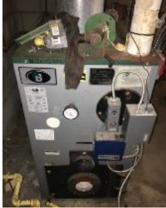
Image 15. Hot Water Boiler
