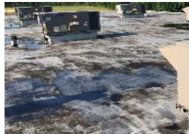
Image 3. Picture of the Building's Roof
