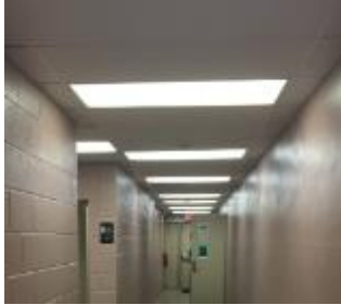
Image 5. Fluorescent T8 Fixtures in Corridors
