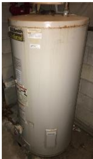
Image 16. Domestic Hot Water Heater
