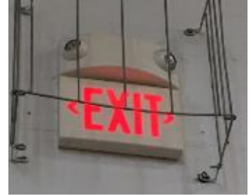
Image 7. LED Exit Sign
