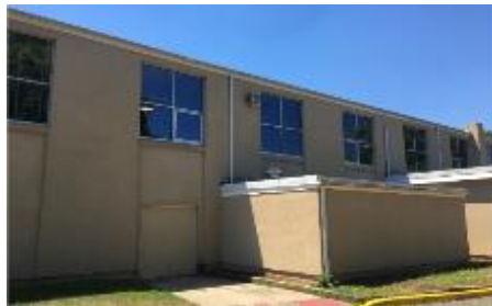
Image 2. Picture of the Building's Exterior Walls & Windows
