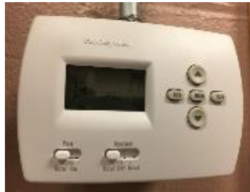
Image 14. Thermostat Inside Maintenance Office
