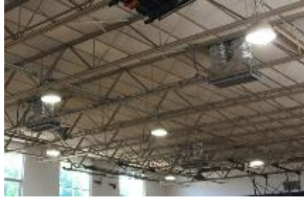
Image 6. Gym High Bay Fixtures
