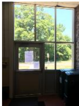
Image 4. Picture of Exterior Door and Window
