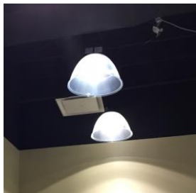
Image 12. Metal Halide Fixtures
