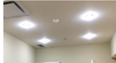
Image 7. Ceiling Mounted Downlights in Restrooms
