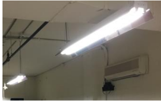
Image 5. Hanging Linear Fluorescent Fixtures
