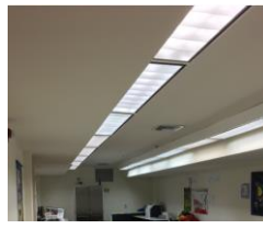
Image 9. Recessed Fluorescent Fixtures
