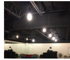
Image 10. Dance Room Lighting Fixtures
