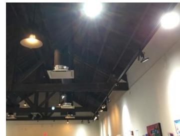
Image 13. Spot Light and Downlight Fixtures in Arts Room
