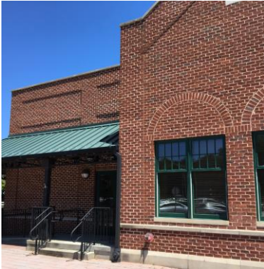
Image 2. Building Exterior Walls
