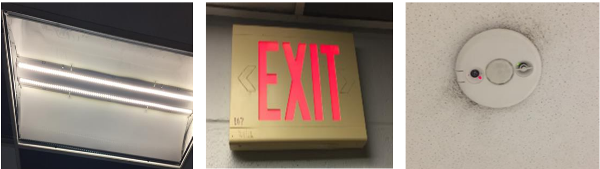
Image 6: LED Tubes Exit Sign & Ceiling Mounted Occupancy Sensors
