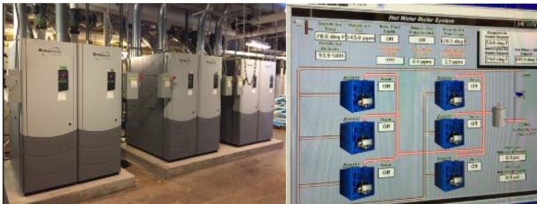
Image 8: Condensing Hot Water Boilers and the BEMS
