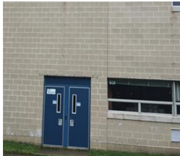
Image 3: Exterior Wall & Door
