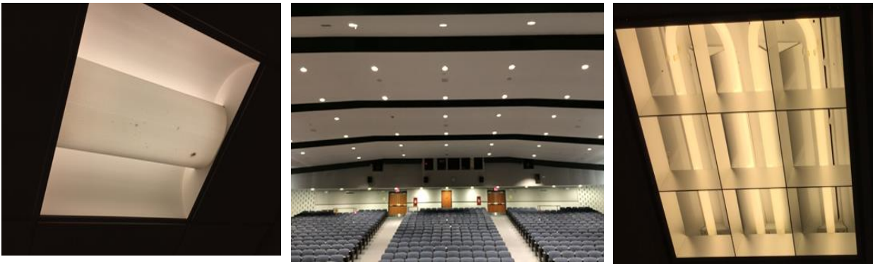
Image 5: Various Interior Lighting System
