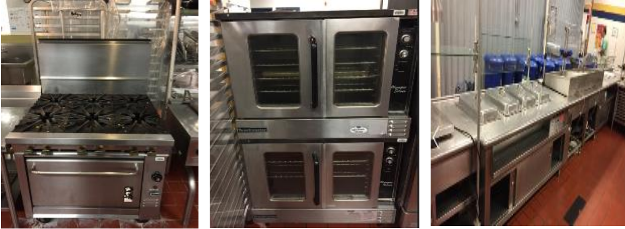
Image 13: Kitchen Gas Cooking Equipment and Warmers
