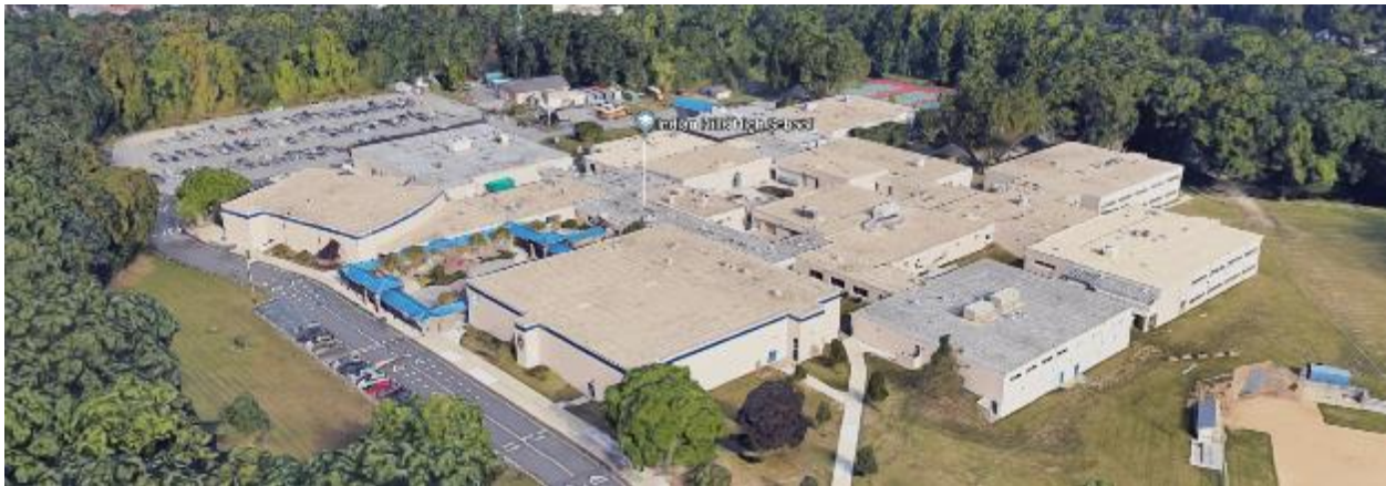
Image 4: Facility Aerial View
