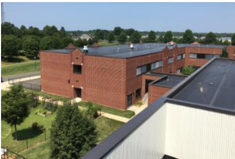
Building Exterior and Roof
