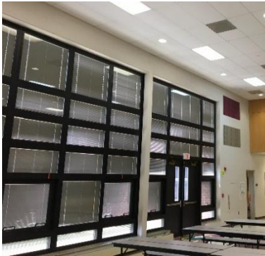
Exterior Door and Windows
