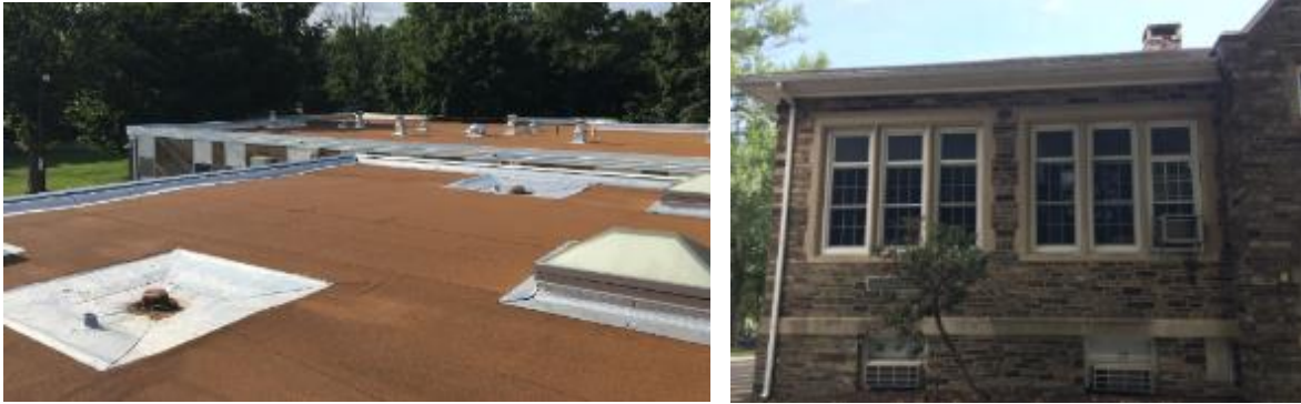
Figure 7 – Building Exterior and Roof
