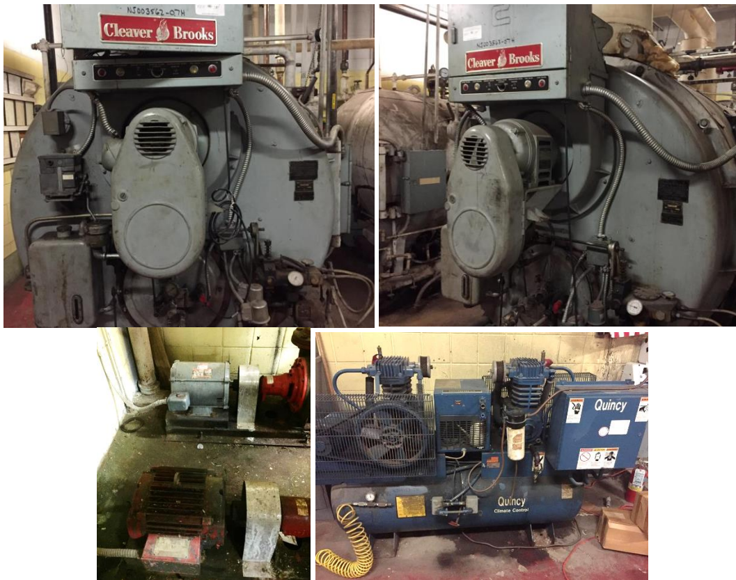
Image 3: Main Boilers, Hot Water Pumps, and Air Compressor (for pneumatic controls)
