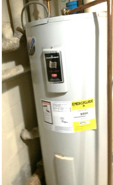
Image 4: Domestic Hot Water Heater
