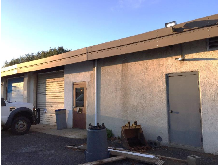
Image 1: Maintenance Building - Front Exterior
