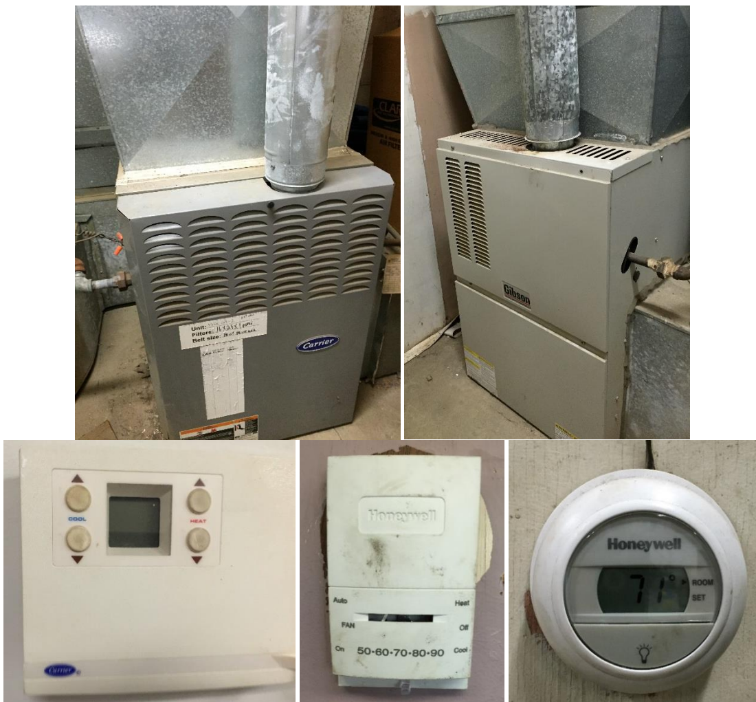
Image 3: Building Heating and Cooling Units and Controls
