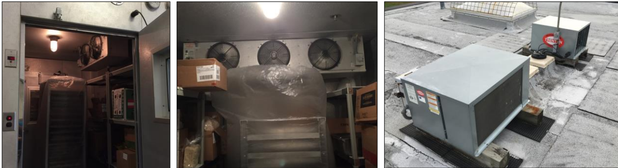
Image Group 10 - Walk-In Cooler & Freezer with Roof Condensing Units
