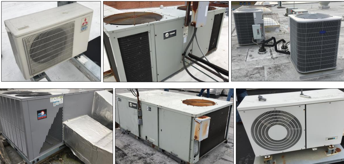
Image Group 6 – Various DX Cooling Systems
