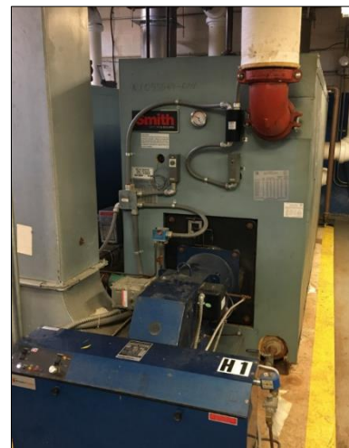
Image 4 - H.B. Smith Hot Water Boiler – 1 of 3
