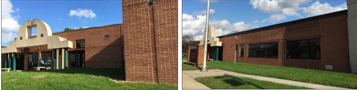
Image Group 1 - Building Envelope
