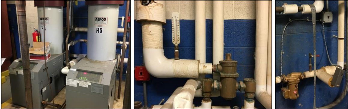
Image Group 8 - DHW Boilers, Mixing Valve, & Recirculation Pump
