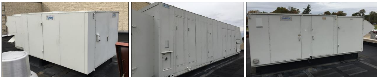
Image Group 5 - AAON Air Handler Units
