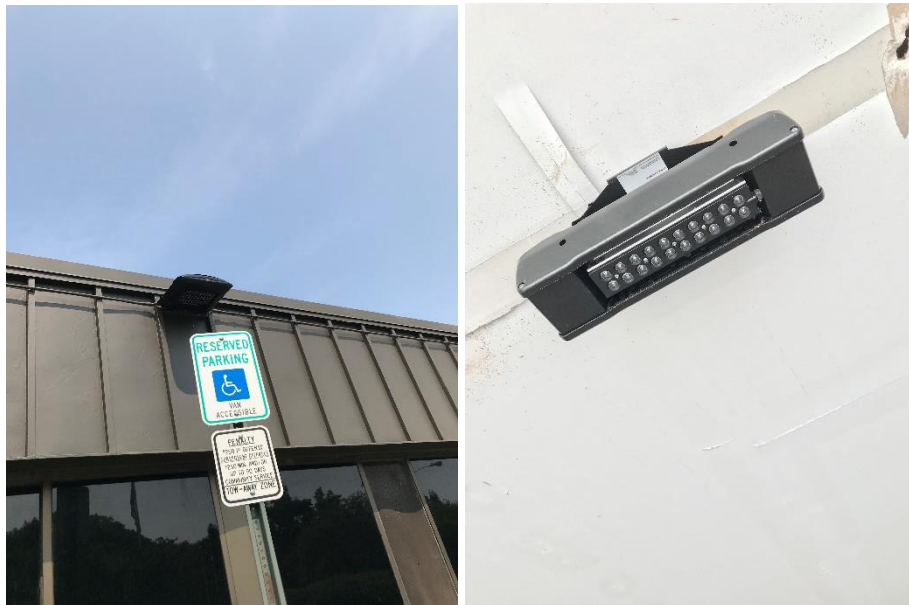
Image 3 Exterior LED Fixtures
