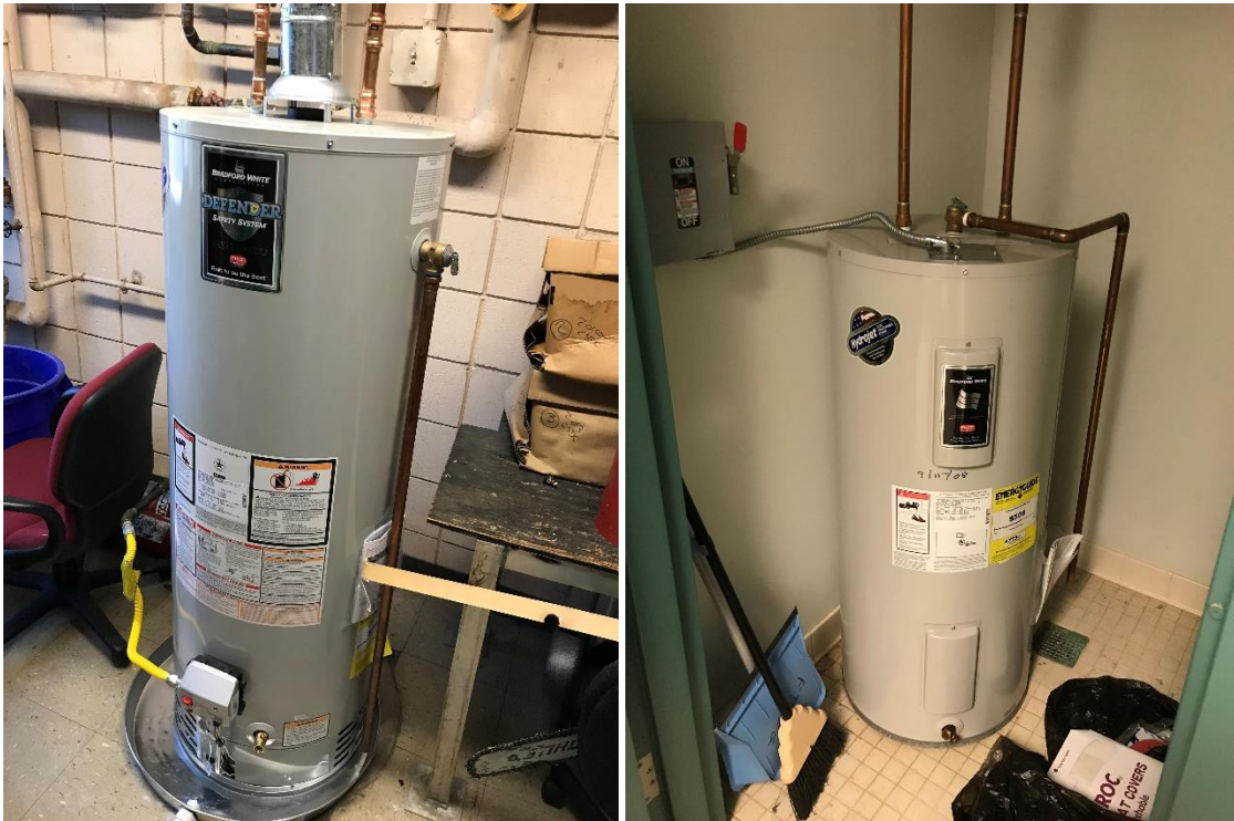
Image 6 Domestic hot water heaters
