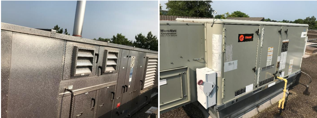
Image 4 Roof Top Units
