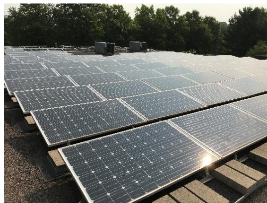
Image 2 Existing Solar Plant on Roof
