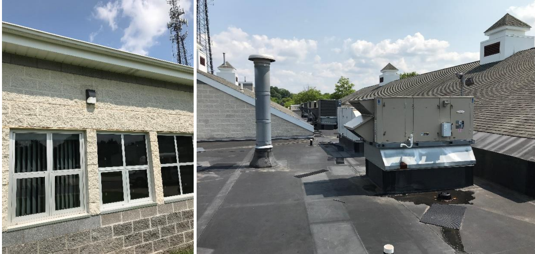
Image 1 Building Exterior and Roof
