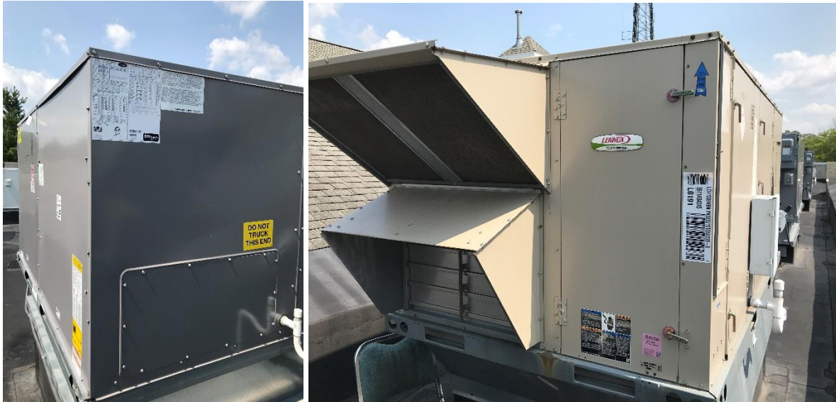
Image 4 Packaged Units on Roof
