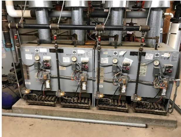
Image 3 Hot Water Boiler System
