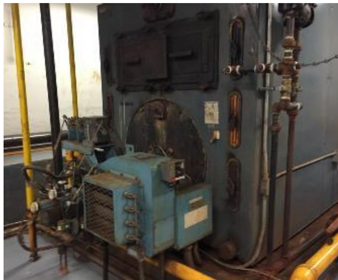
Image 3: HVAC at Buzz Aldrin Middle School
