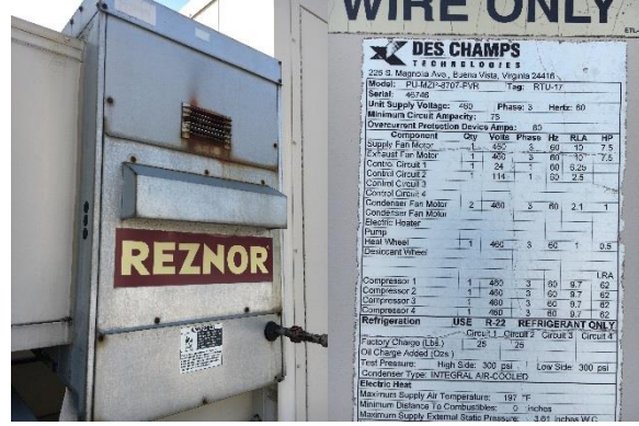
Nameplate for ERU with Air Cooled Integral Condenser and Gas Heater
