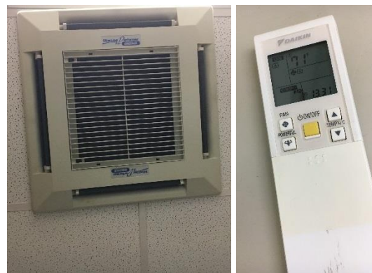
Split HP System – Indoor Unit & Remote Control
