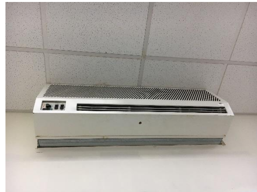
Split AC Systems – Indoor Units
