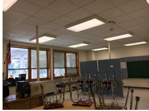
Surface Mounted Box Fixtures
