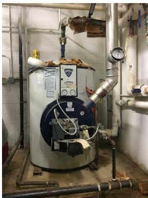
Storage Tank Water Heater
