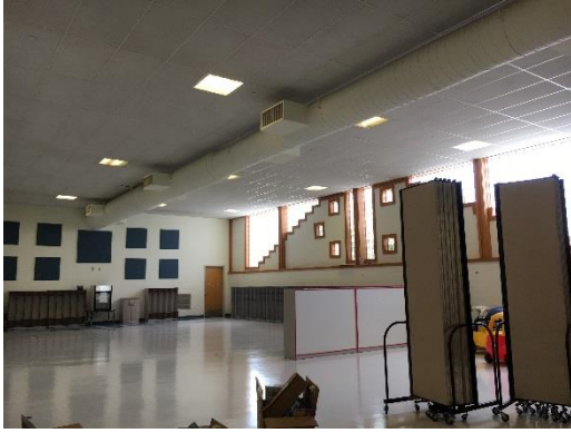
Multipurpose Room Lighting
