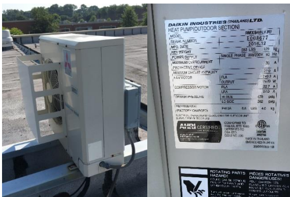
Split HP System – Outdoor Condensing Unit
