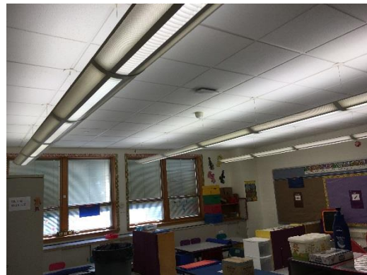
Continuous Row Up Light Fixtures
