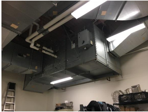
AHU with HW Coil
