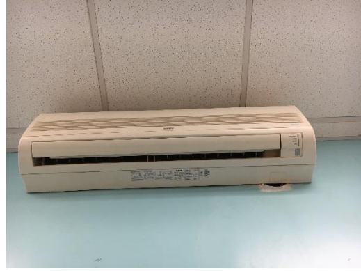
Split AC Systems – Indoor Units
