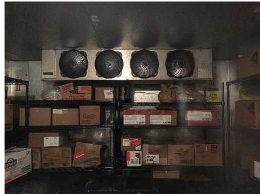
Walk-in Refrigeration Evaporator
