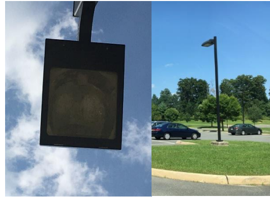
HID Shoe Box Pole Mounted Fixtures
