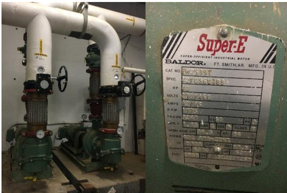
Hot Water Pumps and Motor Nameplate
