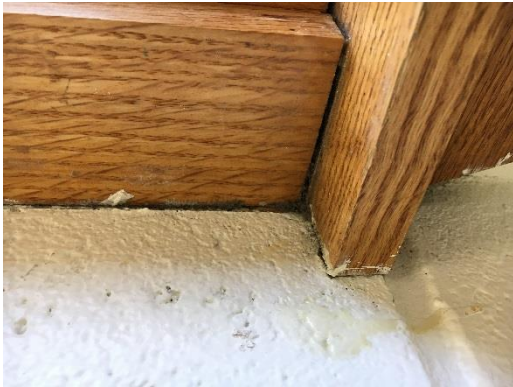
Wooden Window Frame with no Seal
