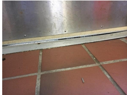
Exterior Door with worn Weather-Stripping
