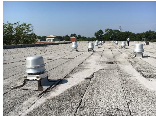
General Building Exhaust
