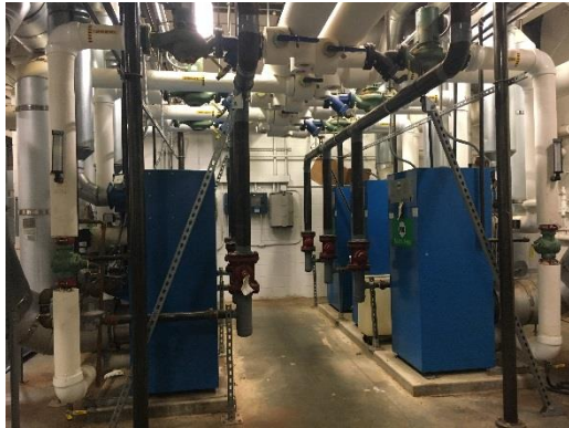
Condensing Hot Water Boilers
