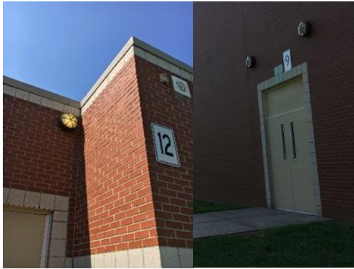
CFL Wall Pack Fixtures
