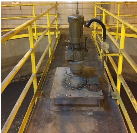
Figure 10 – Grit Vortex Paddle Motor
