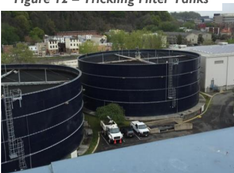
Figure 12 – Trickling Filter Tanks
