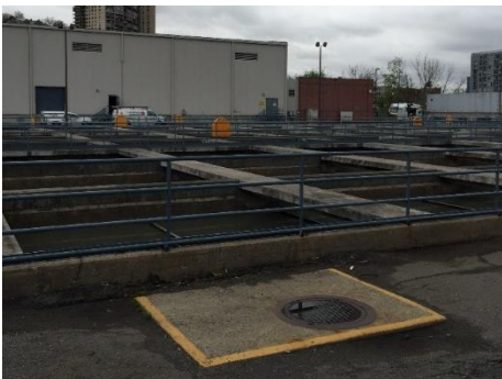
Figure 12 – Trickling Filter Tanks
