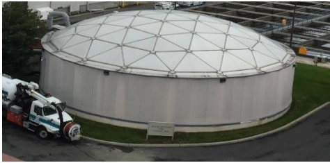
Figure 14 – Sludge Holding Tank
