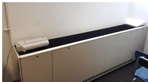
Image 6: Classroom Unit Ventilator
