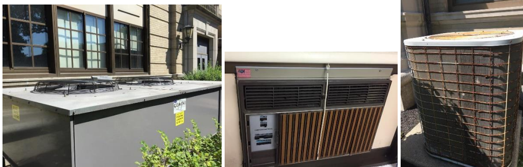
Image 7: Air Conditioning Units
