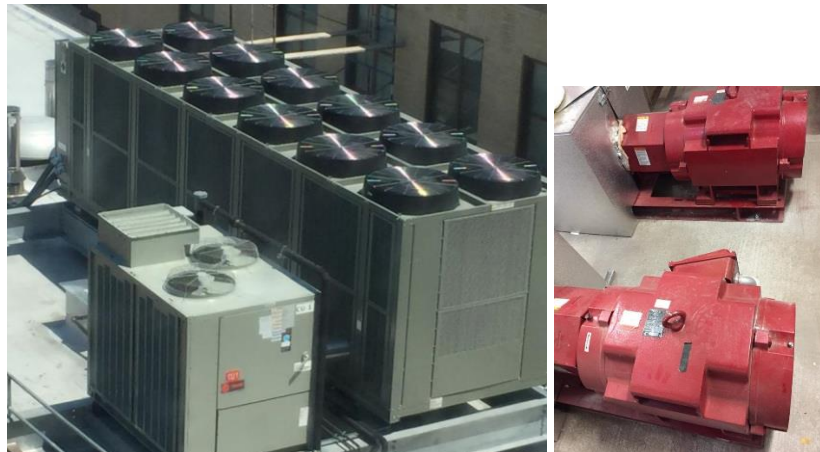
Image 4: Air-Cooled Chiller and Chilled Water Pumps
