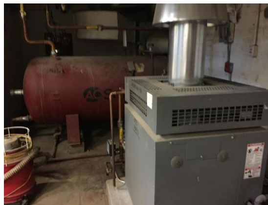
Image 8: Domestic Hot Water Heater and Storage Tank
