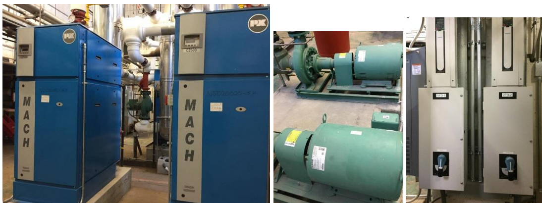
Image 5: New High Efficiency Modular Boilers and Hot Water Pumps with VFDs
