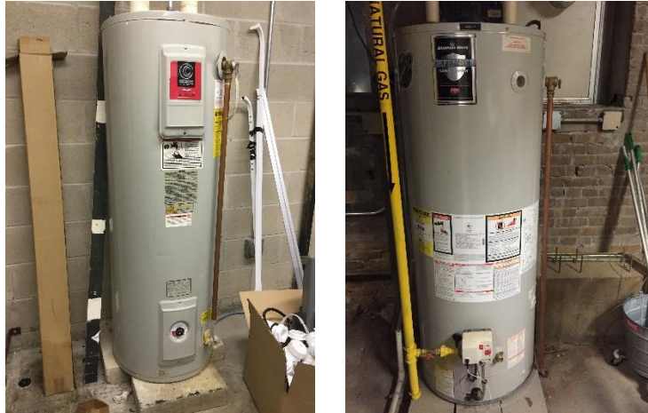
Image 5: Domestic hot water heaters
