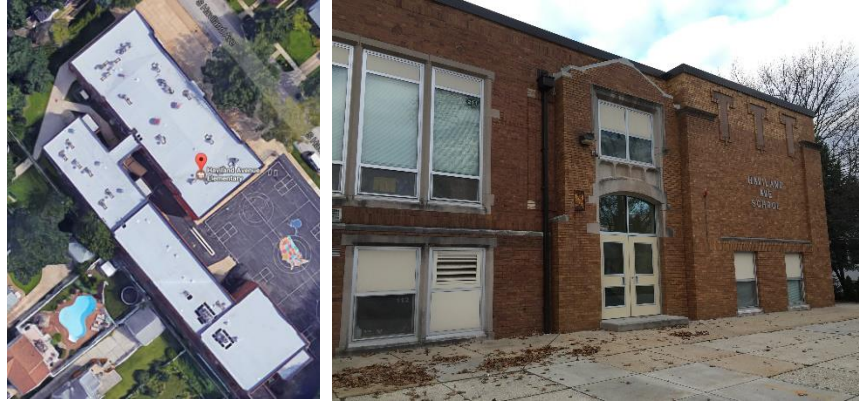
Image 1: Building roof and envelope
