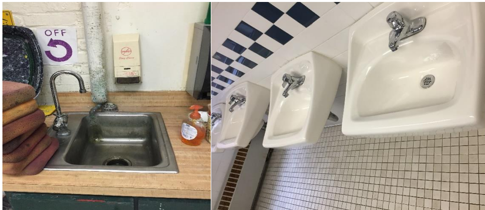
Image 8: Art room sink and restroom sinks
