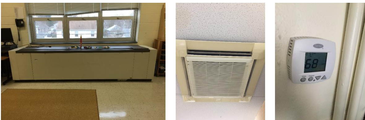
Image 4: Unit ventilators and ceiling cassette units
