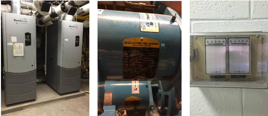
Image 3: Hot water boiler and a sample pump at the mechanical space
