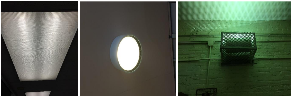
Image 2: Typical lighting fixtures
