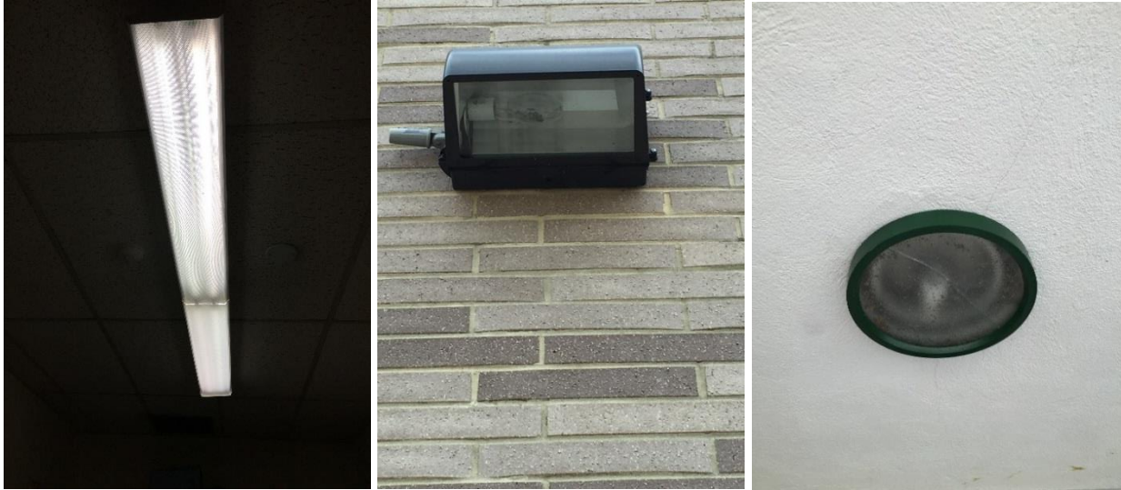
Image 2 Typical lighting fixtures
