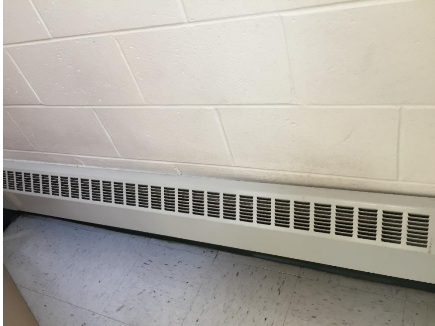
Image 3 Boilers and terminal heat distribution units
