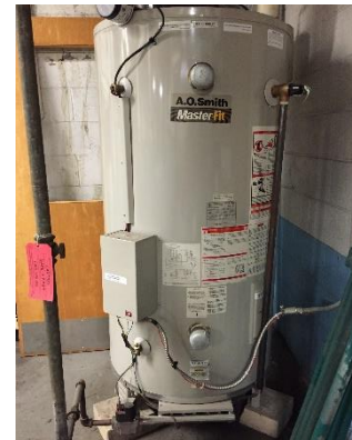
Image 5 Domestic hot water heater
