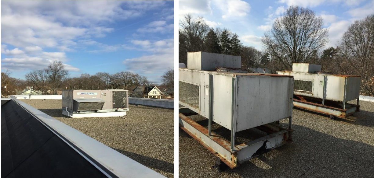
Image 4 Air conditioning equipment
