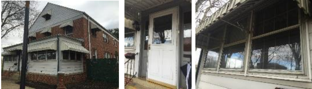
Building Exterior, Doors, and Windows
