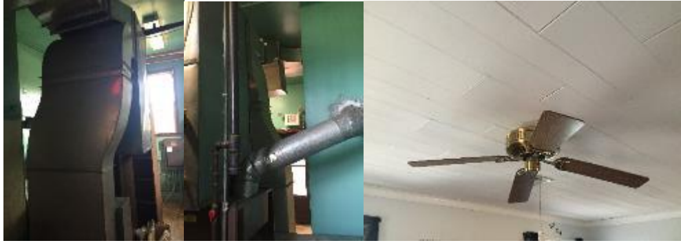
Heating System and Distribution
