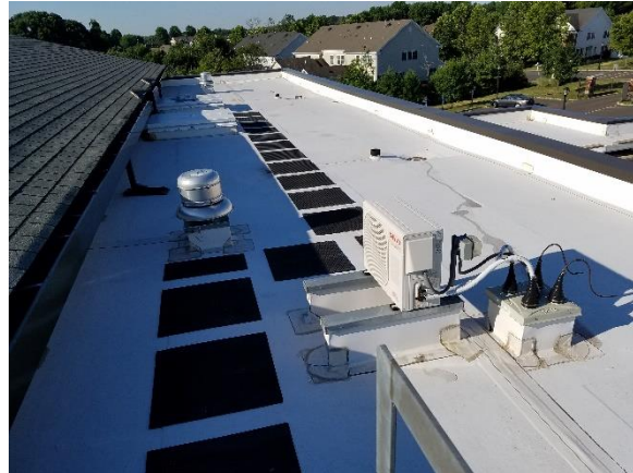
Figure 16 – Ductless Mini-Split
