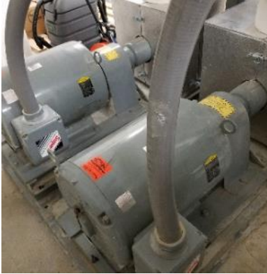
Figure 12 – GSHP Circulation Pumps
