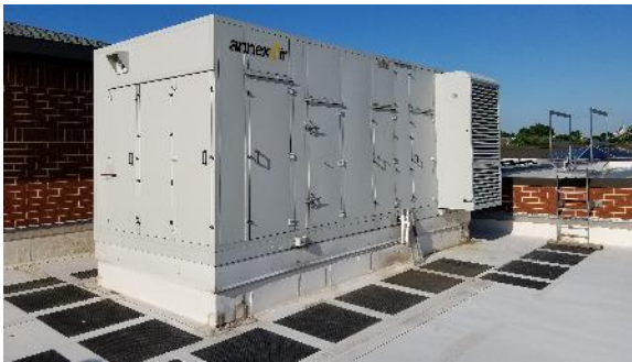
Figure 17 – ERV on Roof
