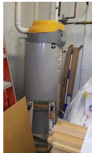
Figure 20 – Kitchen DHW heater
