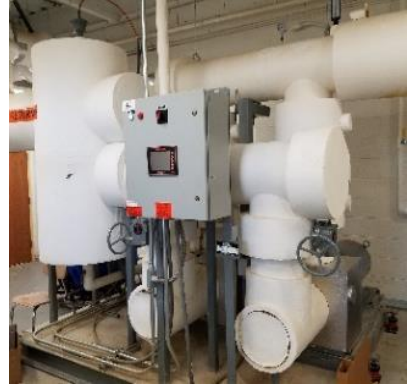
Figure 14 – Pump Variable Speed Drives
