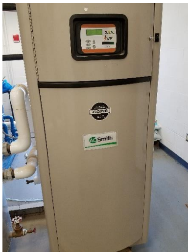
Figure 19 – A.O. Smith Boiler
