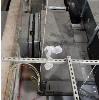
Figure 13 – Water Source HP (in attic over classroom wing)
