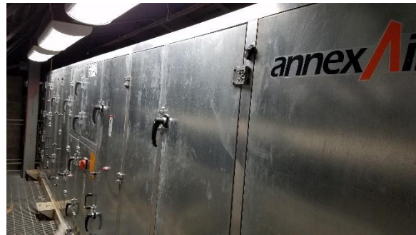
Figure 18 – ERV in Attic
