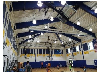
Figure 11 – Gym HID Fixtures
