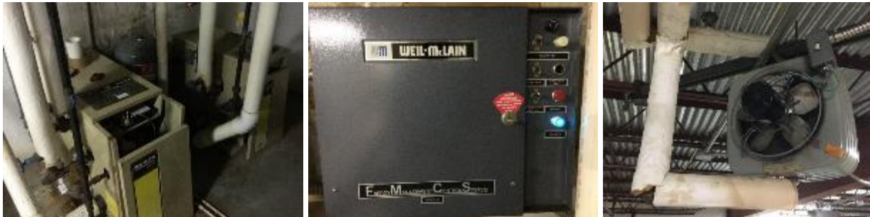
Image 3 – Hot Water Heating System
