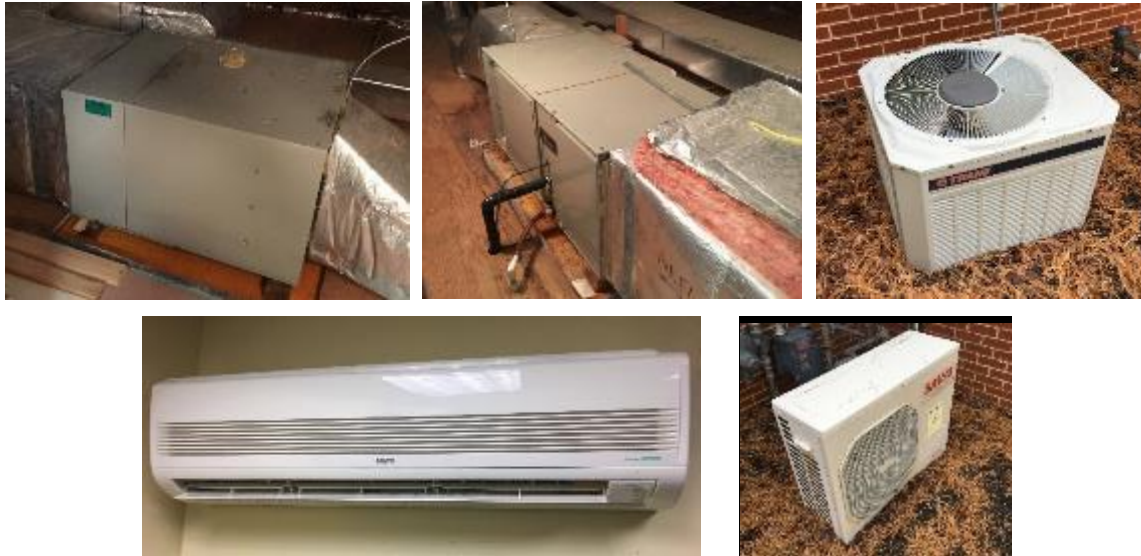
Image 4 – Packaged Furnace and DX Cooling System
