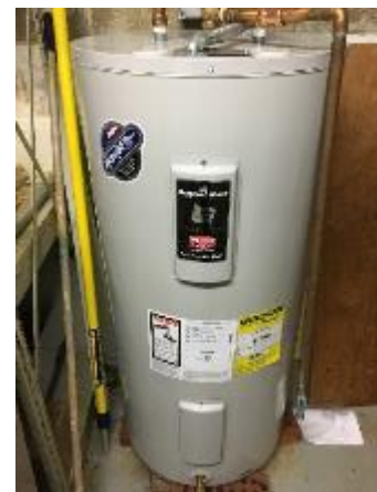
Image 5 – Domestic Hot Water System
