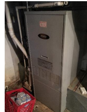
Image 3 - Building Heating System
