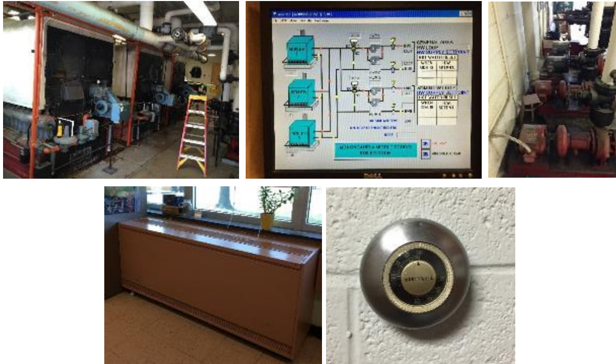
Image 3 Hot Water Heating System
