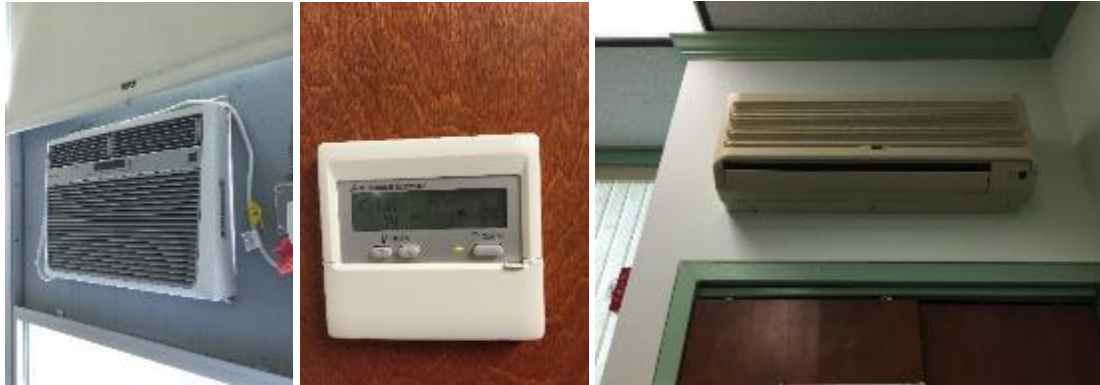
Image 4 Air Conditioning System
