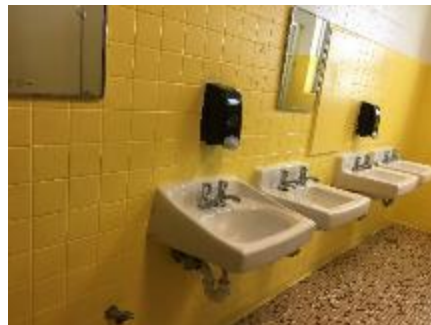
Image 7 Water Using Systems
