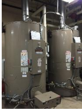
Image 5 – Domestic Hot Water
