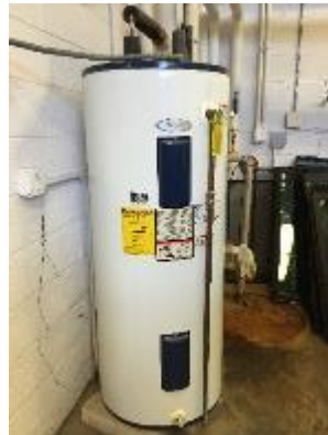
Image 5 Domestic water heating
