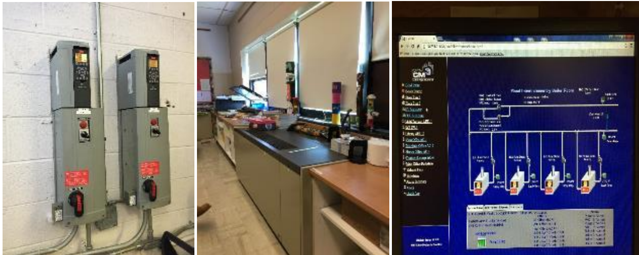
Image 3 Hot water system
