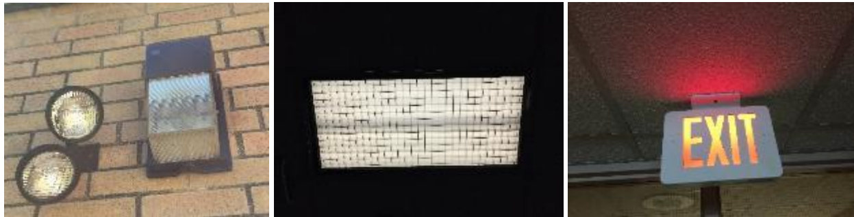
Image 2 Sample of lighting fixtures at the facility
