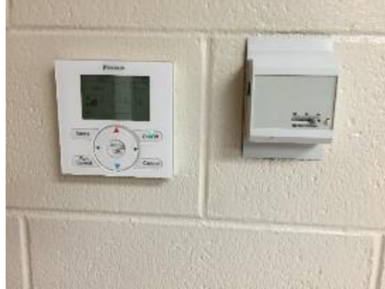
Image 4 Air conditioning system
