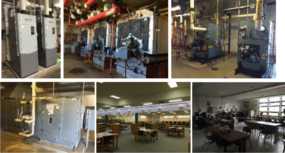
Image 4 Hot Water Heating System
