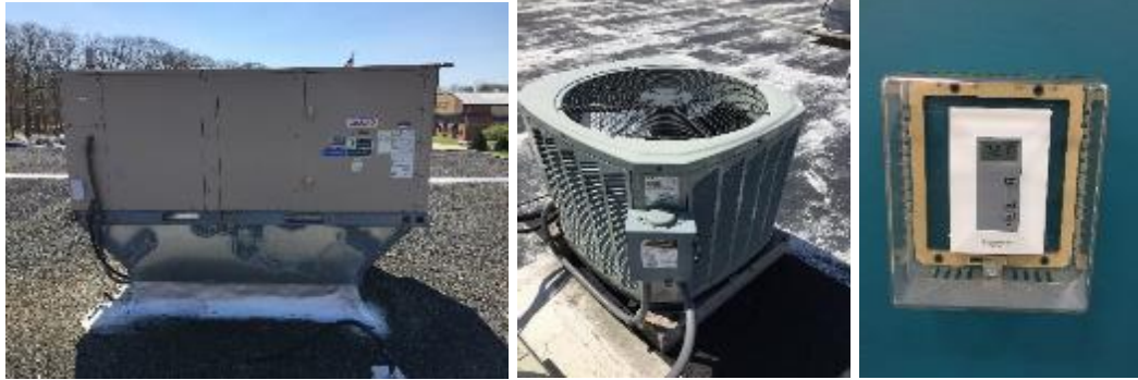
Image 5 Air Conditioning System
