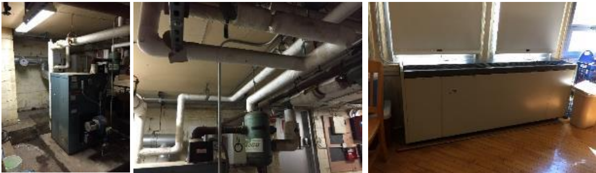
Image 3 Hot water system
