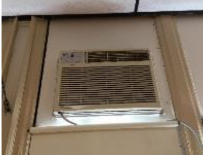
Image 4 Air conditioning system
